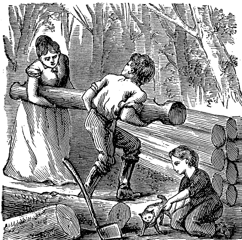
BUILDING THE CABIN-HOME.
